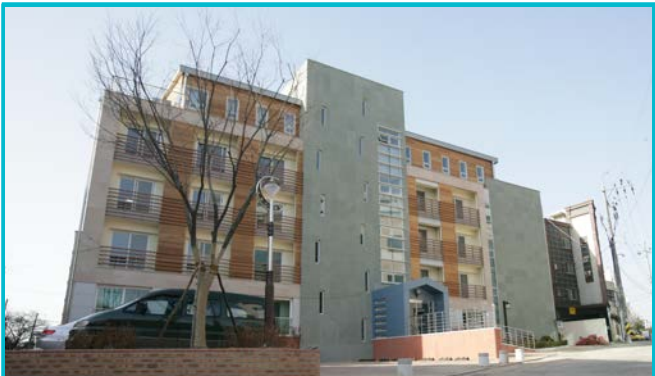
Main Campus Dormitories
